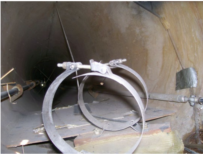
O2 cylinder mount and radio antennas behind.
