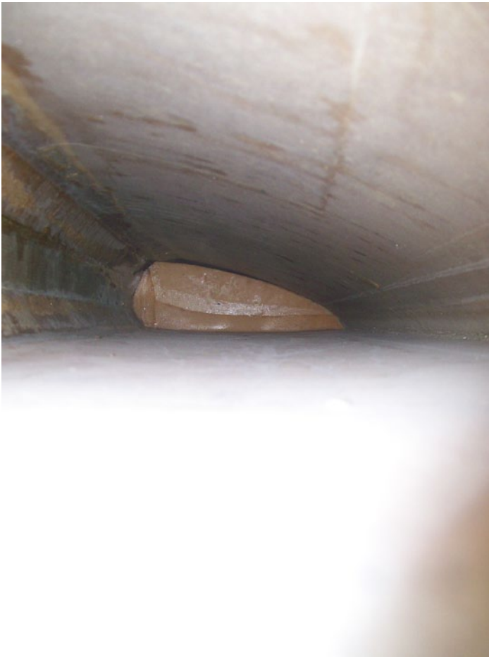
Left wing leading edge D-tube. Note spar cap glue runs talked about in history document.
