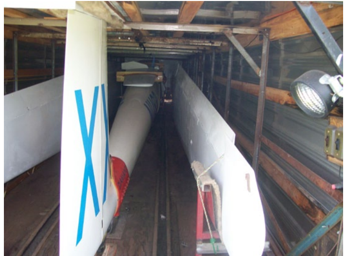
All in its box note the flood light for work in low light conditions.
